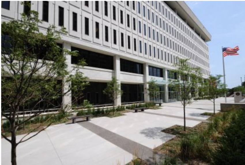
Gerald W. Heaney Federal Building and United States Courthouse and Customhouse, 515 West First Street, Duluth (opened in 1929)
